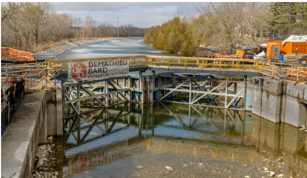
Warsaw Road Swing Bridge in the Trent-Severn Waterway in Ontario.
