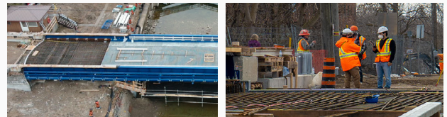
Warsaw Road Swing Bridge during construction.
